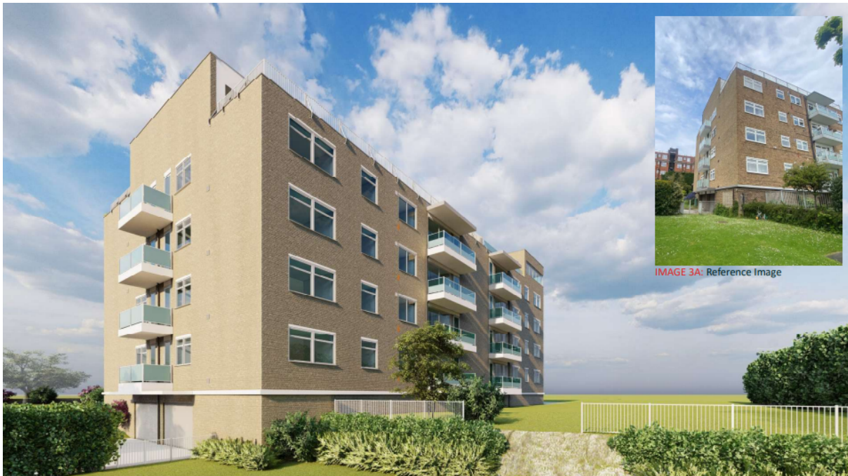
Fig 2 – The existing building from the rear.
